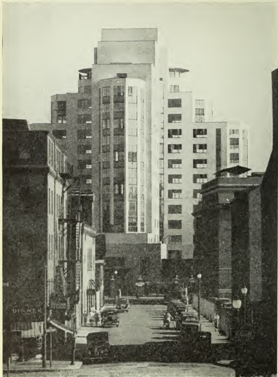
Entrance to George Robert White building from North Grove Street
